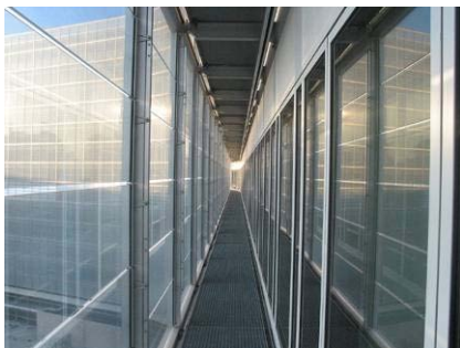
Figure 6-36. View of the large cavity and the louvres in vertical position.
