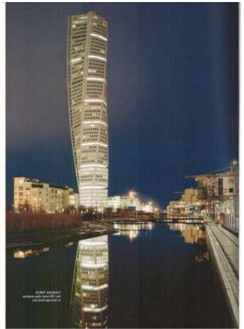
Turning Torso, an apartment building in Malmö, Sweden: all the corridors lit by LED lighting
