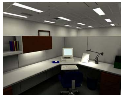
Lower power densities achieved with task/ambient lighting solutions
